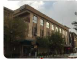
Good condition(Goran hotel)
