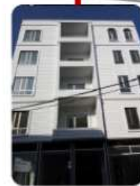
Good condition(Clinic building)
