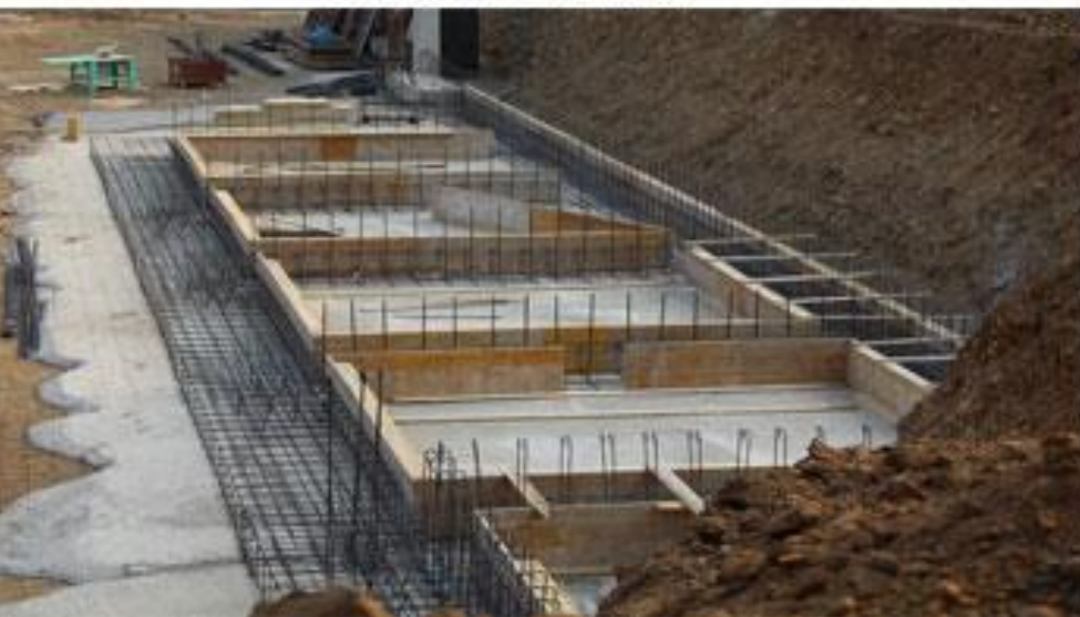
Figure.4: Shallow foundations.
