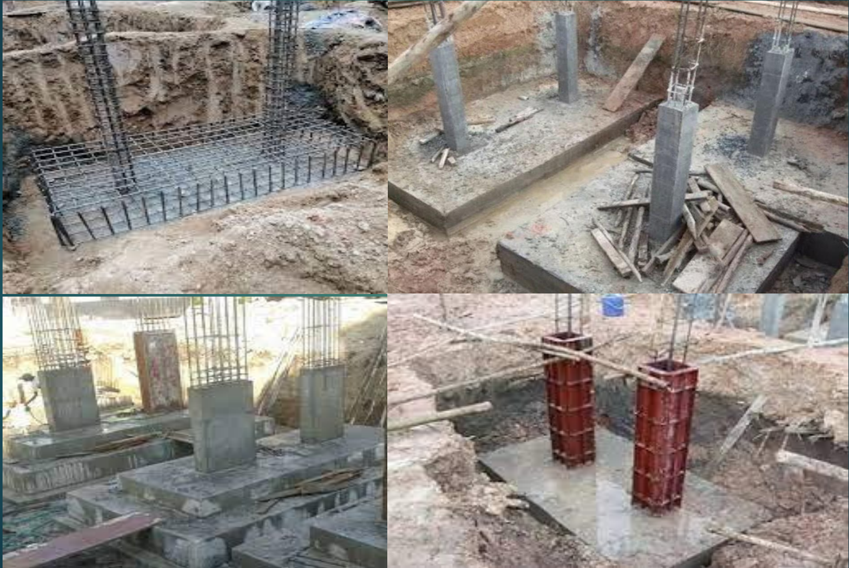
Figure.9: Combined footing.
