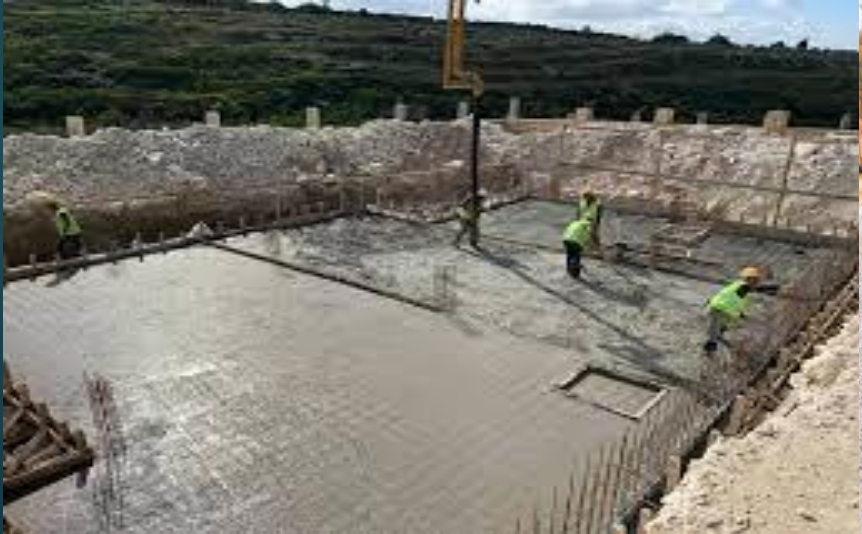
Figure.13: Raft foundation.
