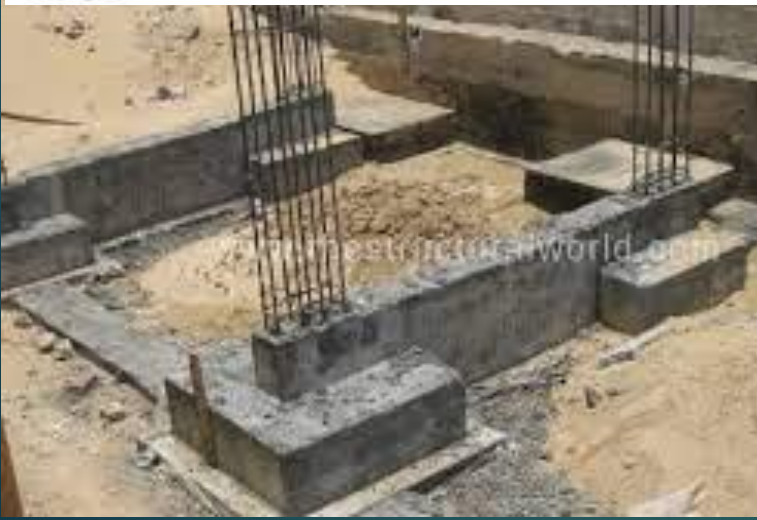
Figure.11: strap footing.
