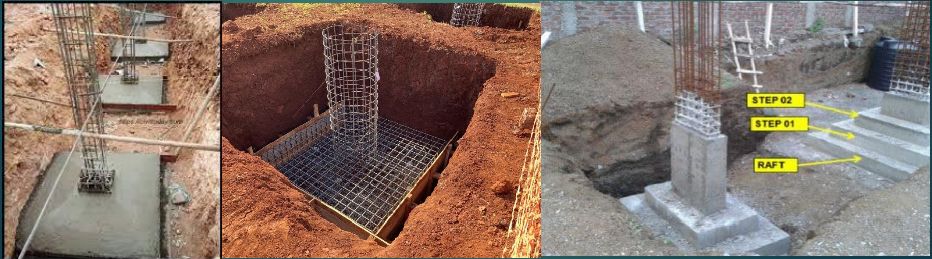
Figure.7: Single column footing.
