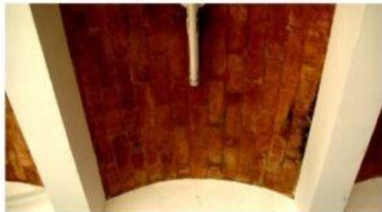
Jack Arch Floor
