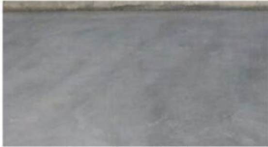
Cement Concrete Floor
