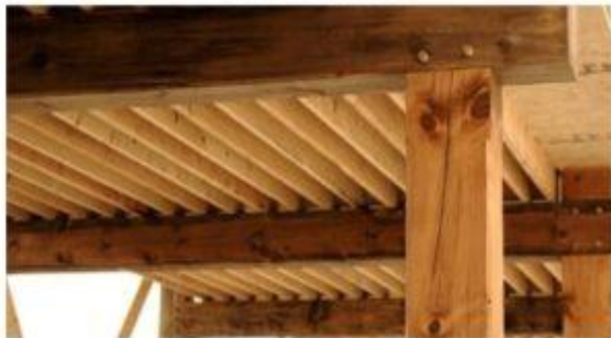
Timber Upper Floor
