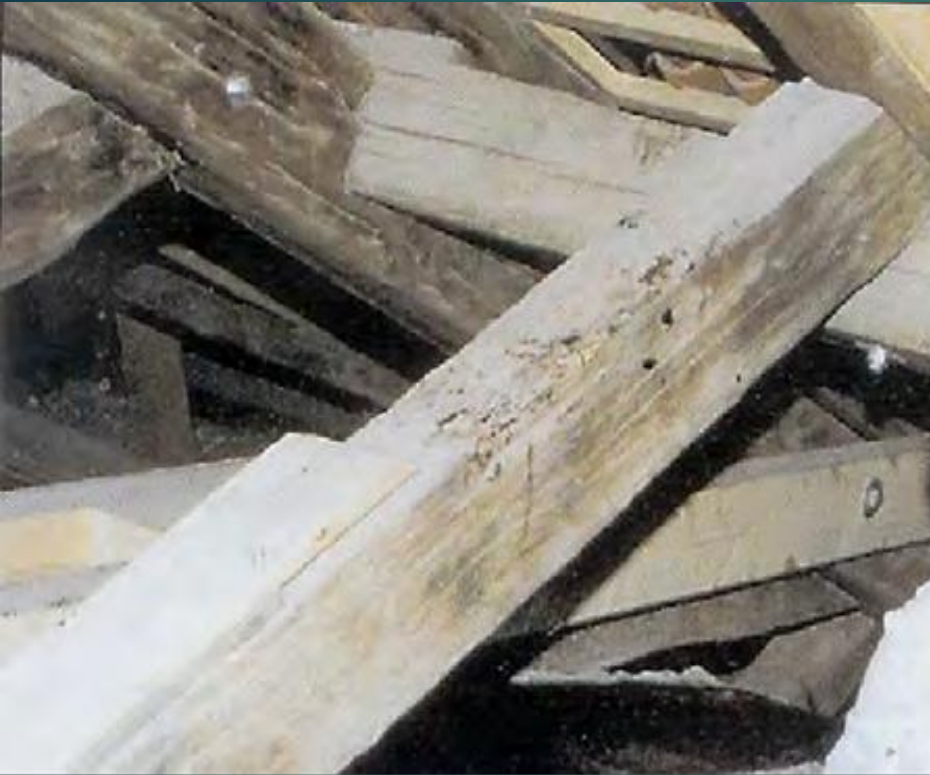
Figure.3 : Timber degradation
