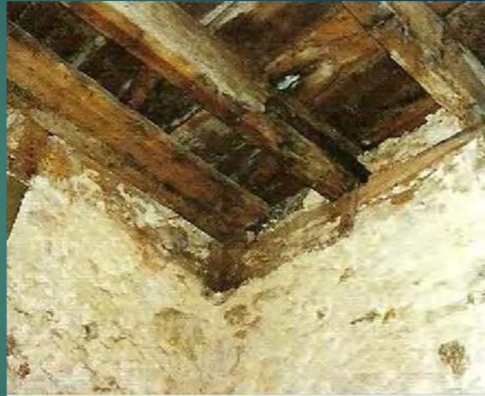
Figure.3 : Timber degradation
