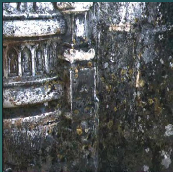
Figure.2: Degradations in stone masonry
