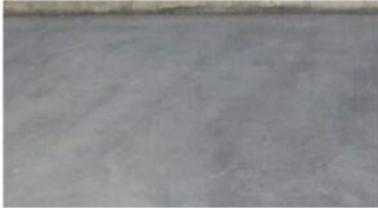
Cement Concrete Floor
