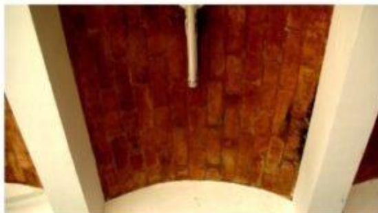
Jack Arch Floor
