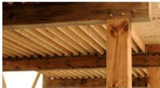
Timber Upper Floor
