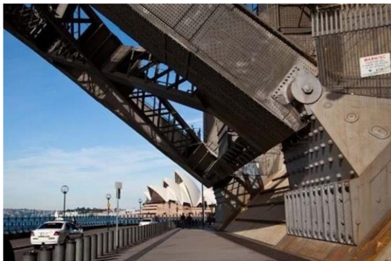
External Pinned support
