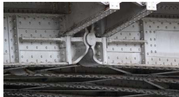
Internal Pinned support
